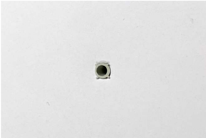
Drill a hole (Ø 6mm) and insert the wall plug.
