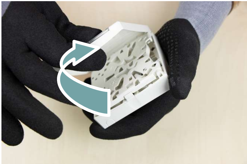
Open the OTO: press the top part of the outlet and remove the lid.
