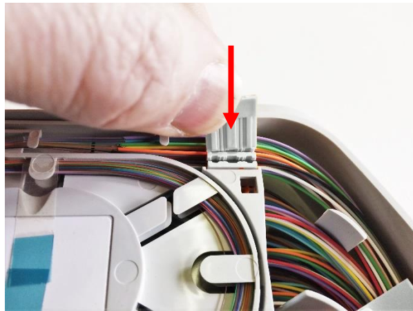
10.7.2 Replace the pigtail for a new one and insert all pigtails back into the 900 \mu holder and push them down with the 900 \mu insertion tool.
