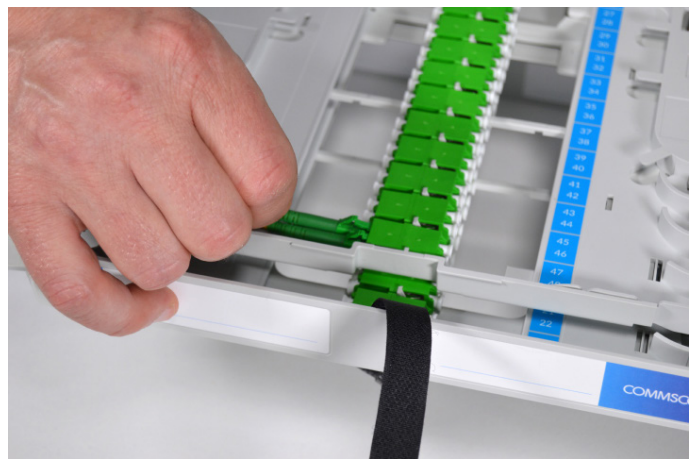
6.4. Remove the velcro and the dust caps. Clean all connectors before patching. Start patching at the bottom (LC as example).
