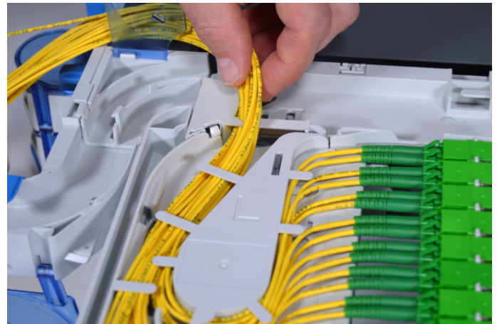
6.7. Carefully guide the patch cords through the channel.
