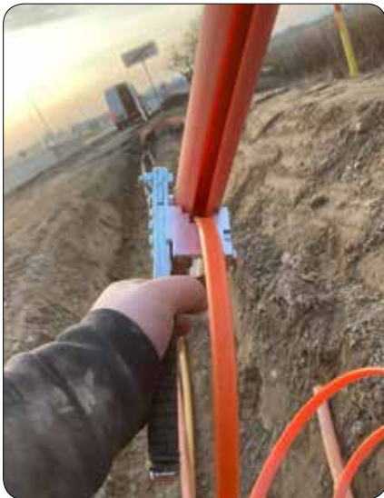
EASY FIBER DUCT SLITTER XL cuts a wide groove in large fiber ducts in a single operation.
