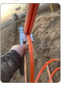
EASY FIBER DUCT SLITTER cuts a wide groove in the most commonly used duct types/ sizes in one operation.
